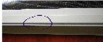
Groove in window around hole cut
